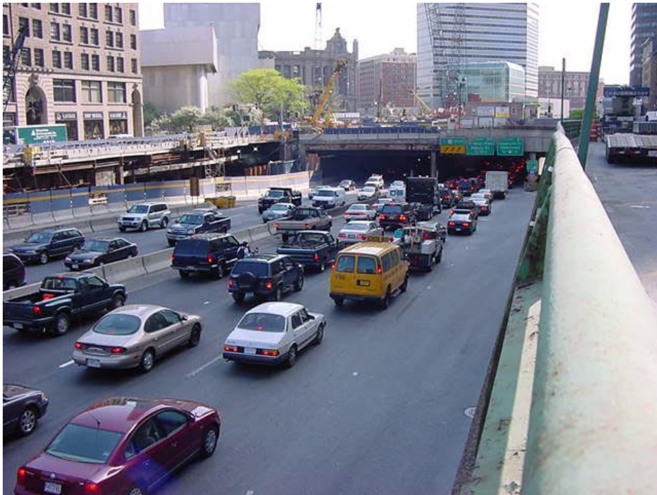
Figure 4-3: A view of the Central Artery.
